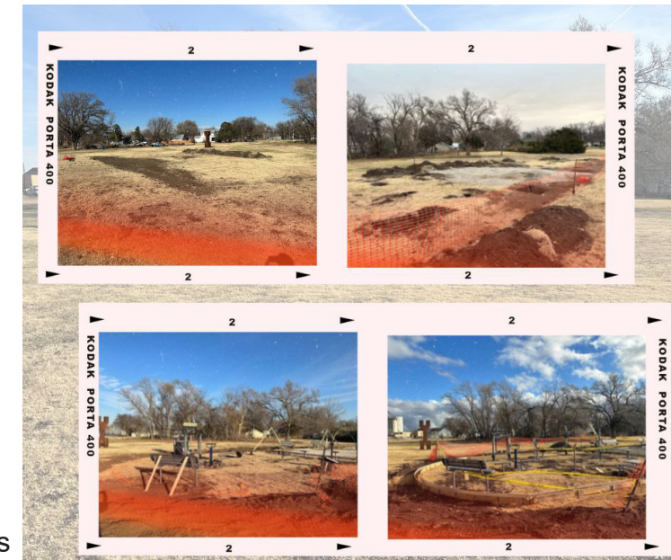
Progress photos from the site.
